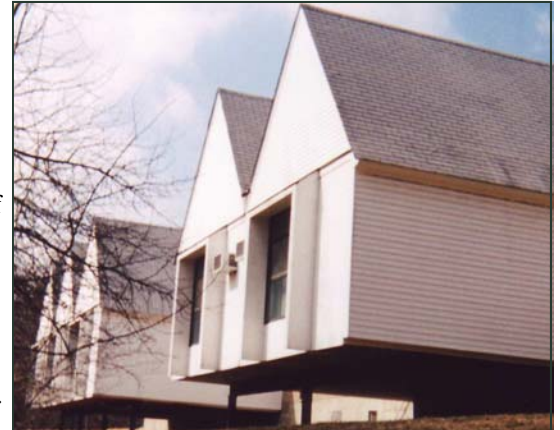
Adding insulation under these Boys and Girls Republic buildings will reduce utility costs and make them more comfortable without changing their appearance.
