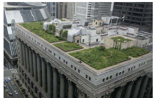
The green roof atop Chicago's City Hall demonstrates the City's commitment to sustainability.
