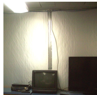
Installed foam insulation (existing) on the windows to prevent excessive air leakage and loss of heat.
