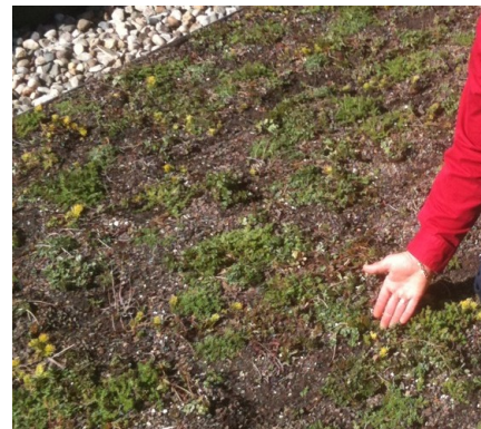
The Green Roof on Warren's Police Headquarters
