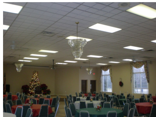
Existing lighting at Lathrup Village City Hall
