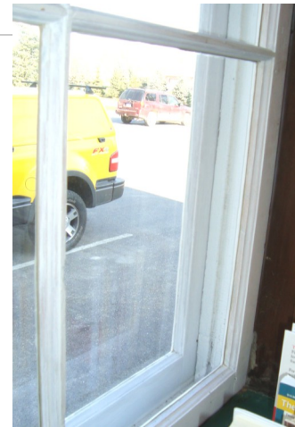
Restored original windows and storm windows installed.
